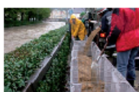
Hesco flood barrier control, Austria.
