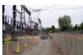
Hesco flood walls protect Walham electricity substation, Gloucester.
