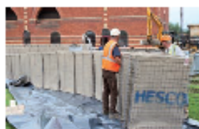
Construction crew extending Hesco units at Mythe water treatment plant in Tewkesbury.
