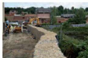
Construction crew fill Hesco units at Mythe water treatment plant in Tewkesbury.
